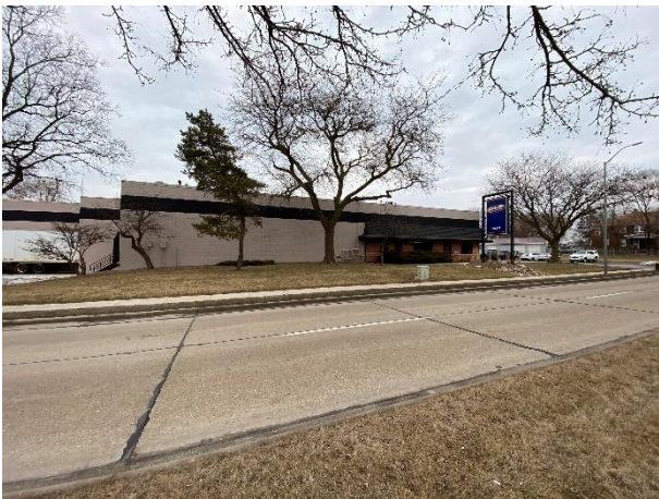
Looking north from the subject property
