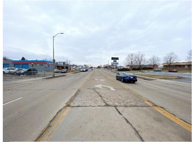
Looking west along Rapids Drive
