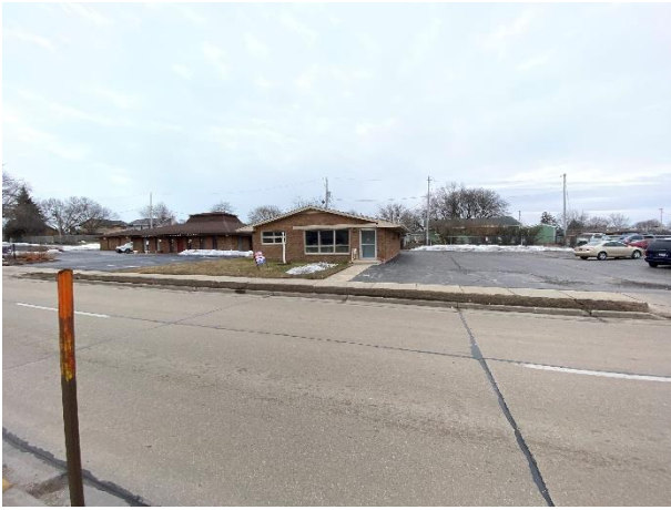
Looking south at the subject property from Rapids Drive
