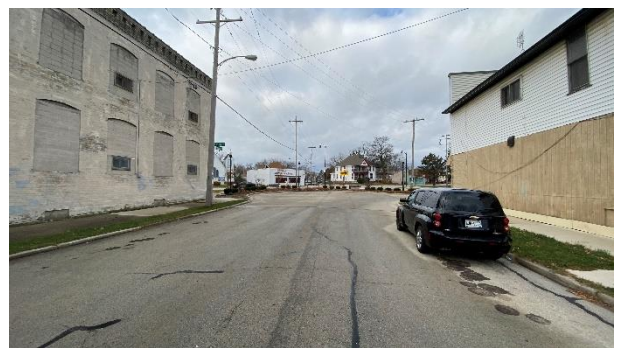
Looking west on Prospect Street
