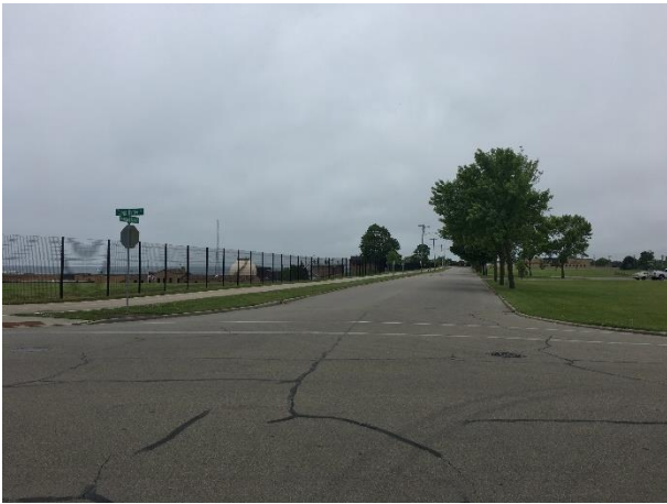
Looking south from 21 st Street down Roosevelt Park Drive
