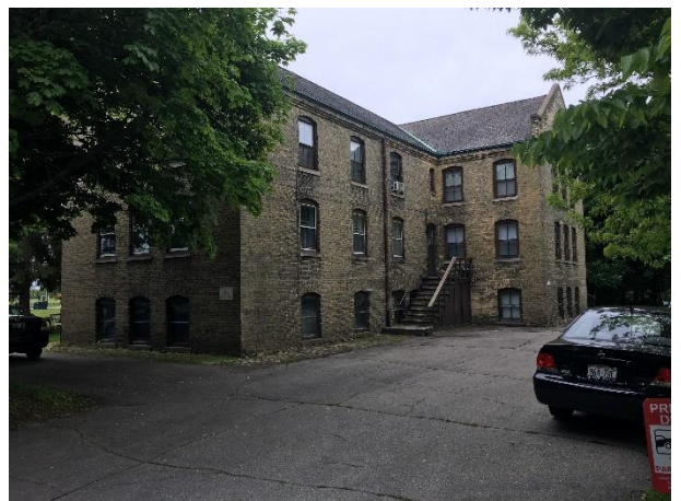
Looking southwest at the gatehouse from the DeKoven Center property
