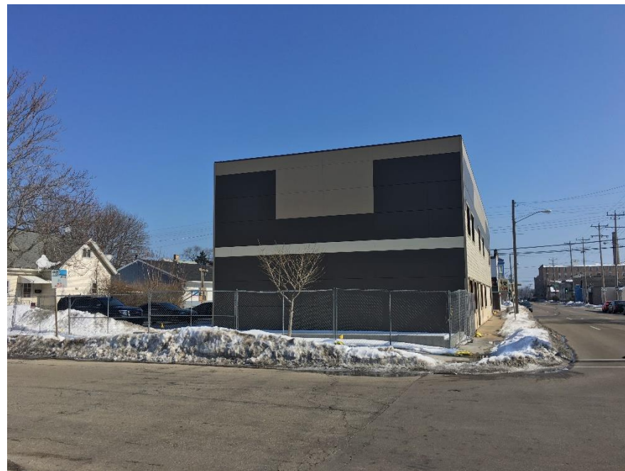
LOOKING AT WEST FAÇADE
