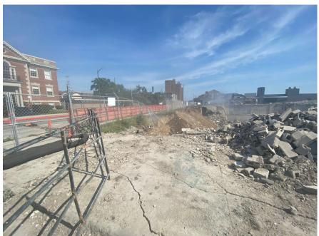
left in place to help stabilize the site and adjacent rightsof-way. Upon demolition of the building's upper floors removal of basement interior walls the walls to remain for stability were observed to unstable and compromised. The intent of leaving the western and southern basement foundation walls in place was to provide stability to adjacent rights of way until the site could be redeveloped.
