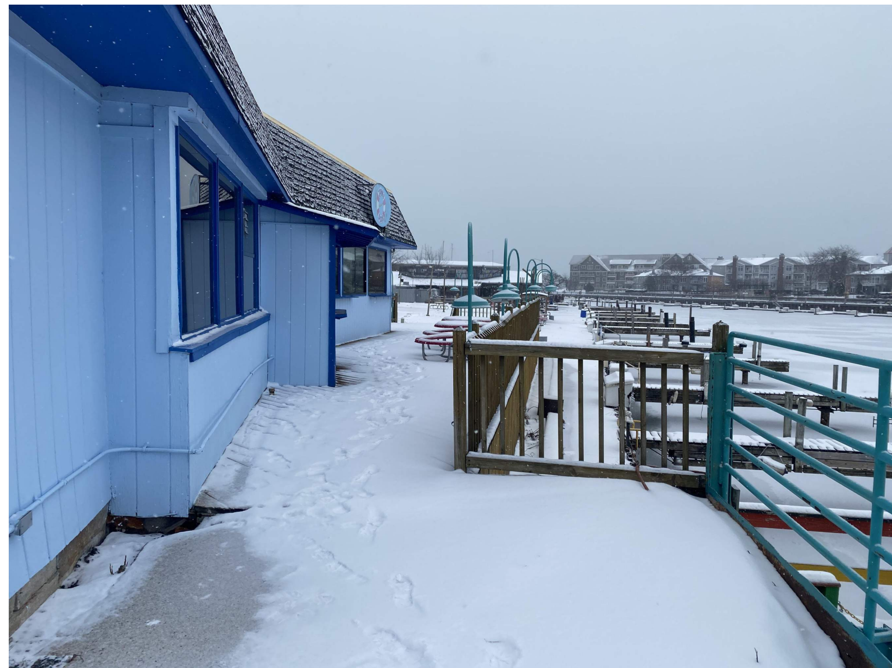
EXISTING BUILDING REAR (SOUTH) FACE
