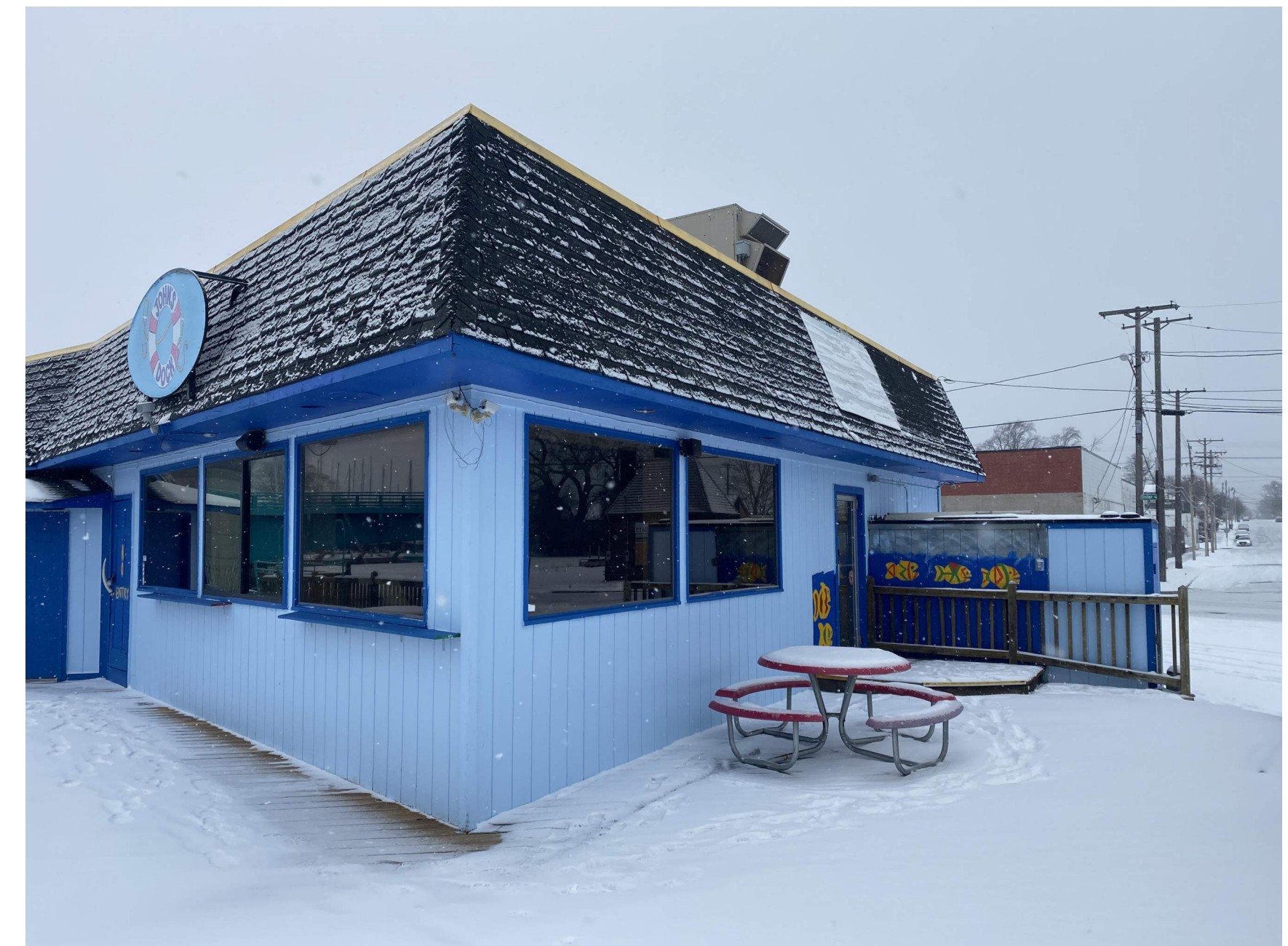
EXISTING BUILDING SE CORNER
