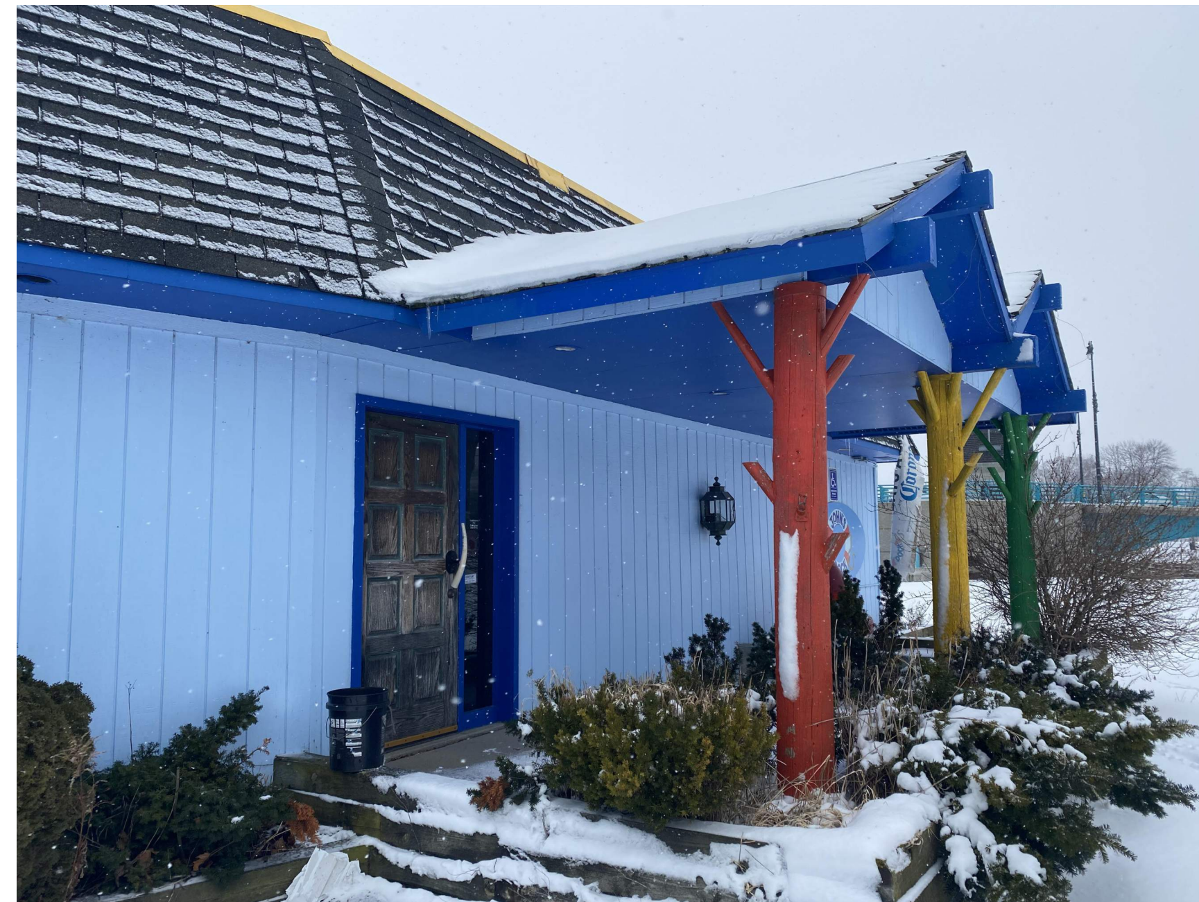
EXISTING BUILDING FRONT (NORTH) ENTRANCE
