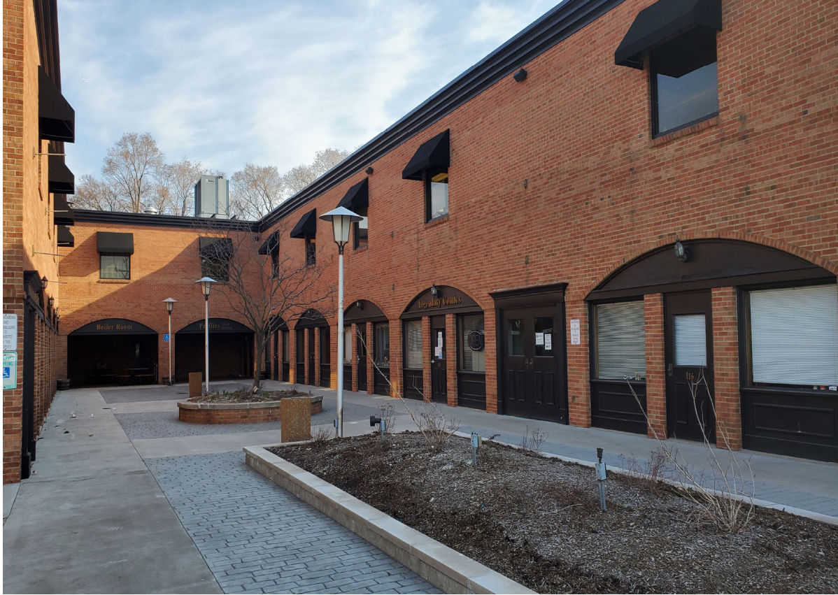
North view from parking lot
