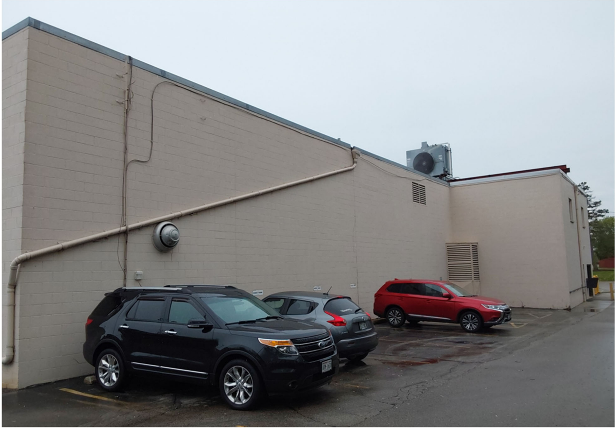
North side ( rear) of building
