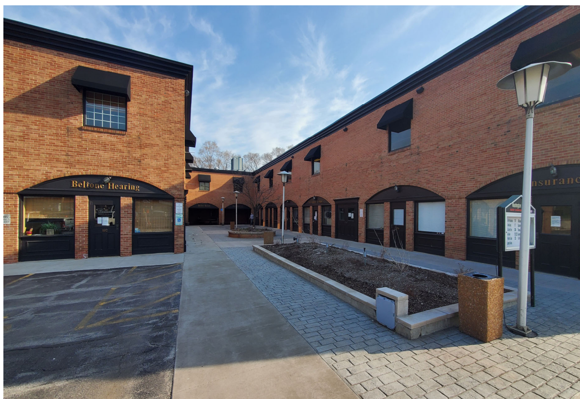
North view from parking lot
