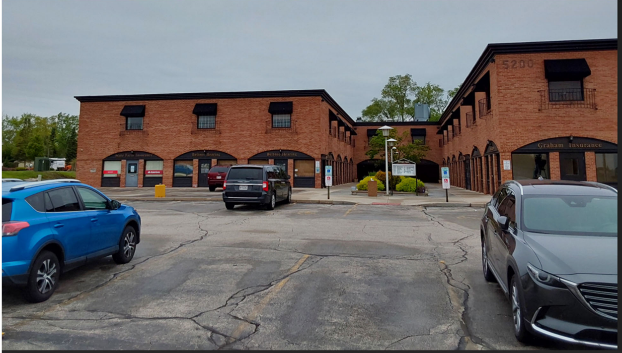
North view looking at building
