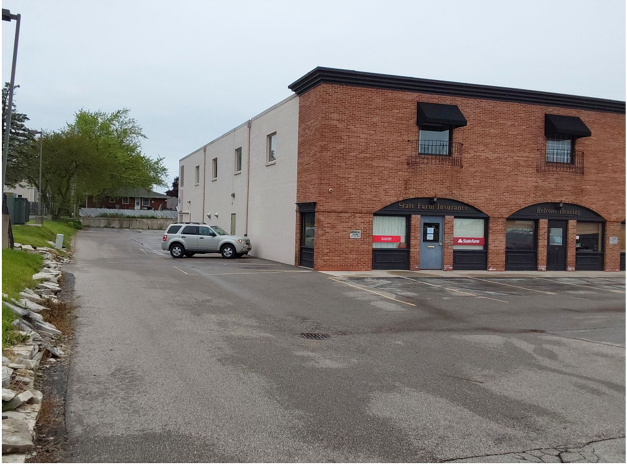
West side- view from parking lot
