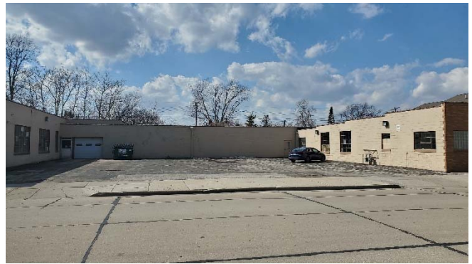
Looking west into parking area
