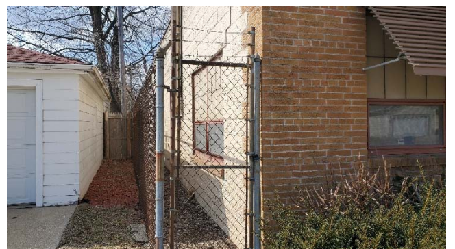
Looking west down south side of building
