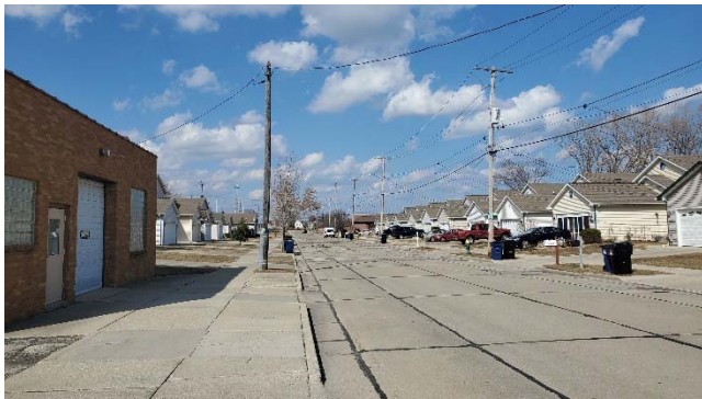
Looking north down Grove
