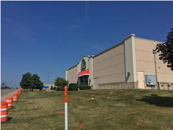
Looking at existing south building façade along Durand Avenue
