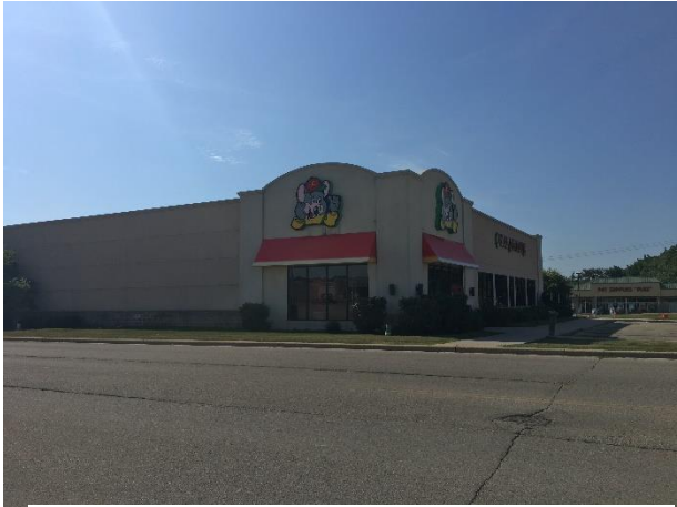
Looking at existing north and west building façades
