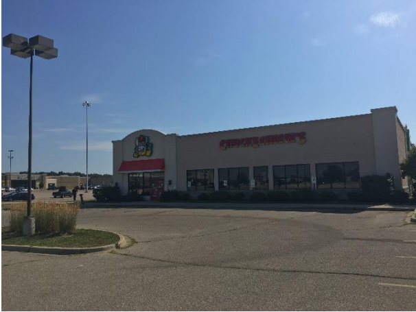
Looking at existing west building façade
