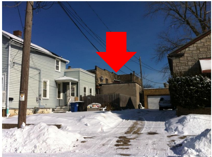
Looking from West to subject property from Superior Street
