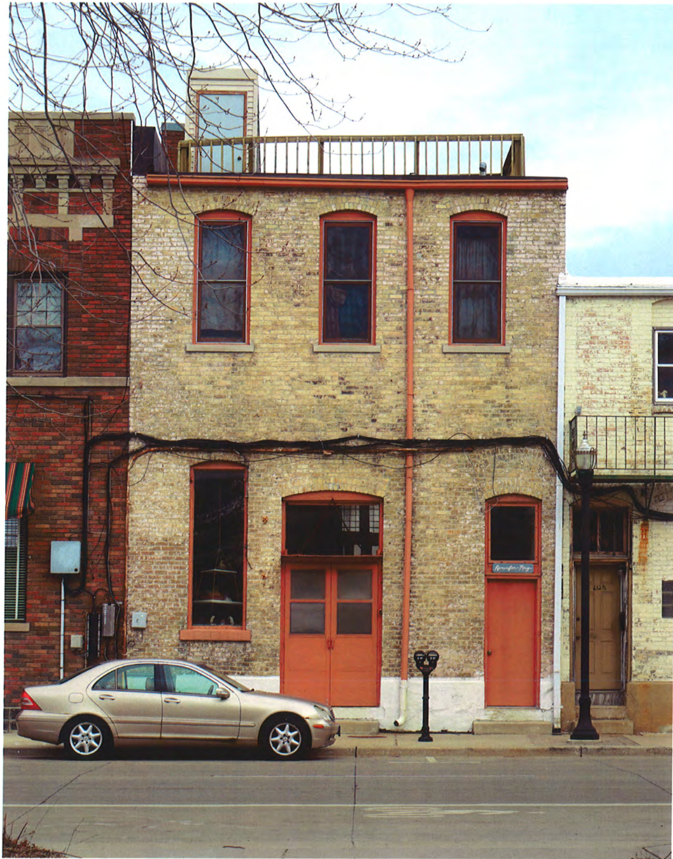
South Elevation- 614 Seventh Street
