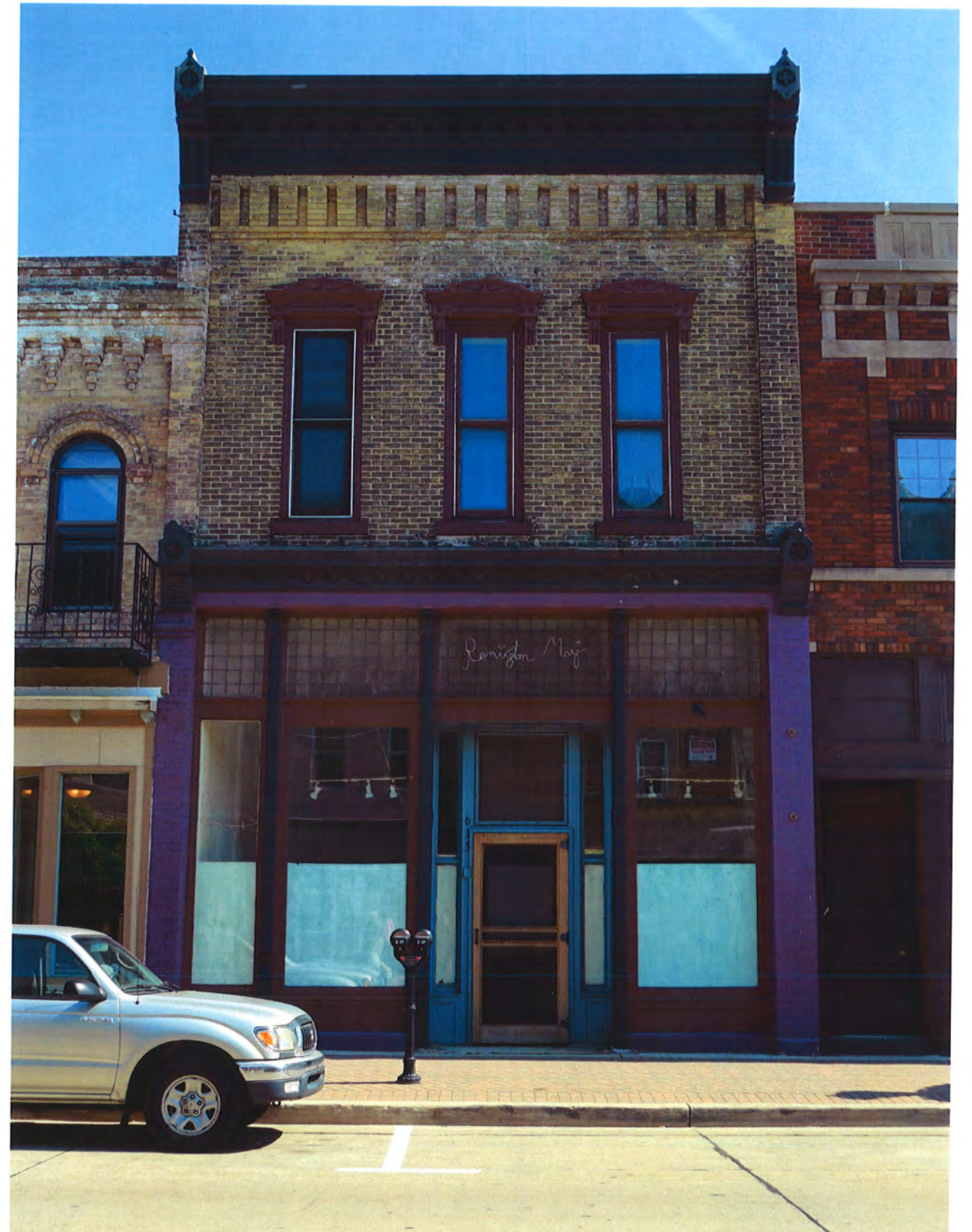
North Elevation- 613 Sixth Street
