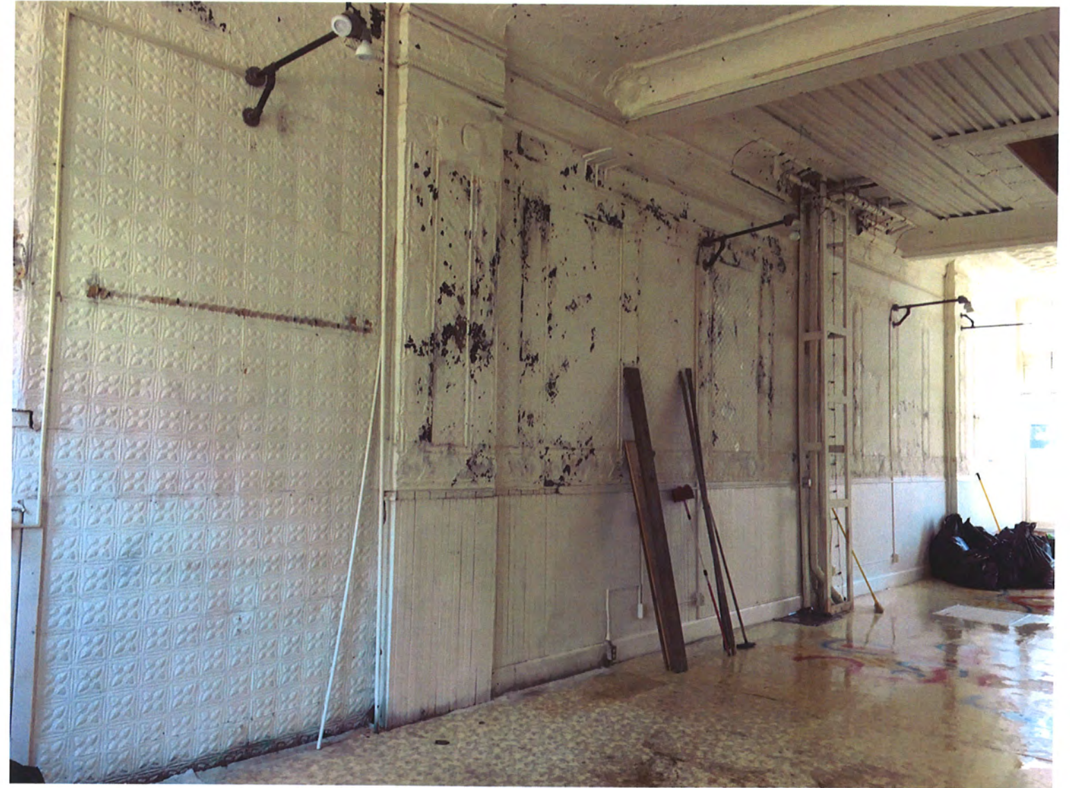
Initial Repair of Tin Ceiling and Walls and Repainting is ongoing.
