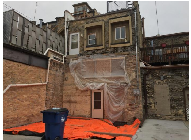
Close up of rear of subject property
