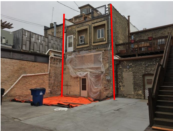
Looking at rear of subject property (red)
