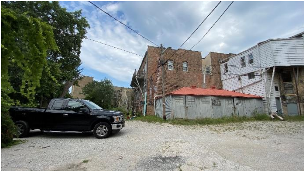
Looking at the rear of the subject property
