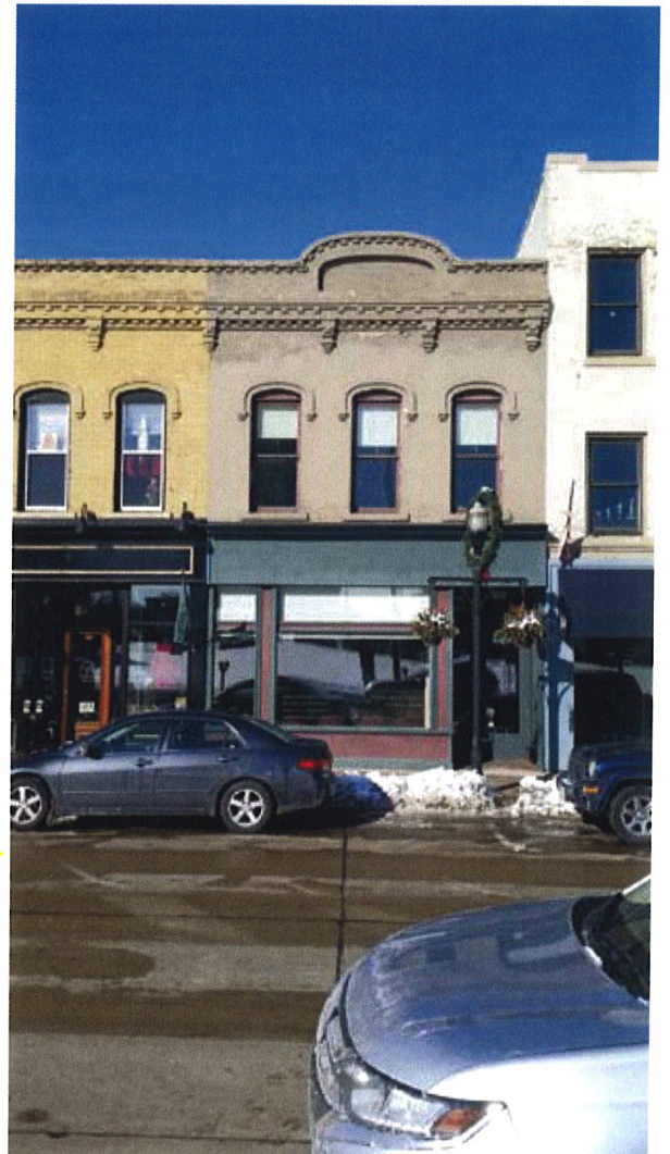
View North - 308 Sixth Street
