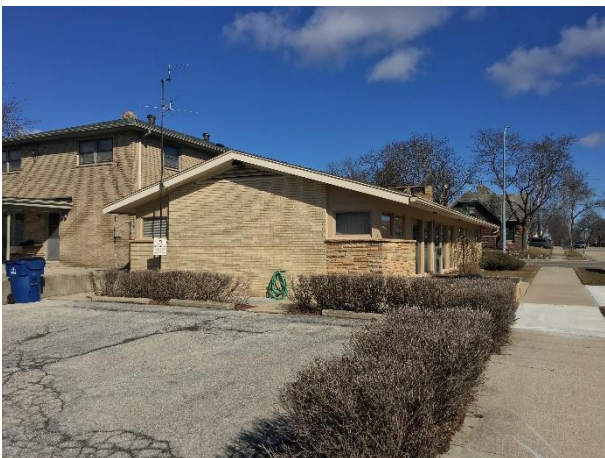
Looking north at rear of subject property
