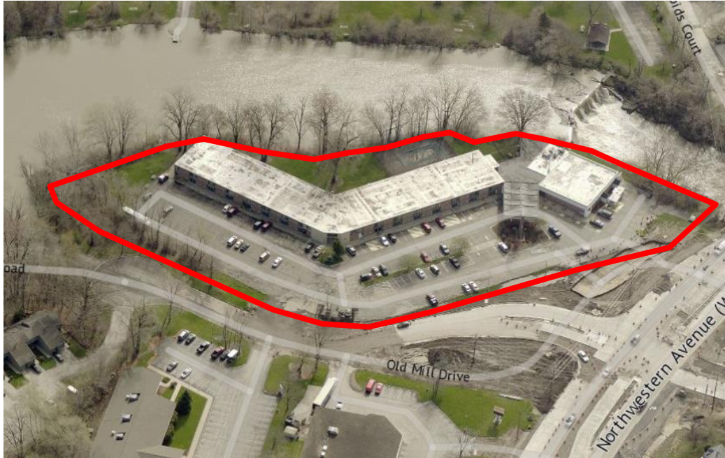
Birdseye view of the property, indicated in red (image from City Pictometry). North is to the left
