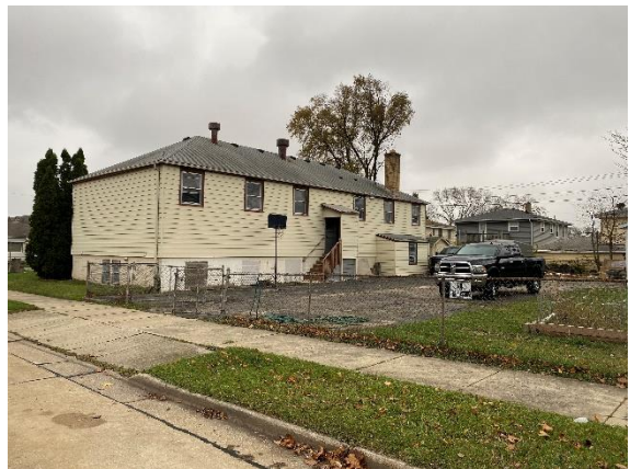
Looking Southeast at rear of building
