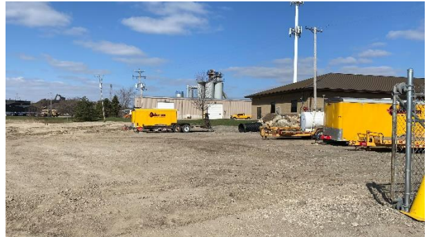
Looking south at site from Oakes Road
