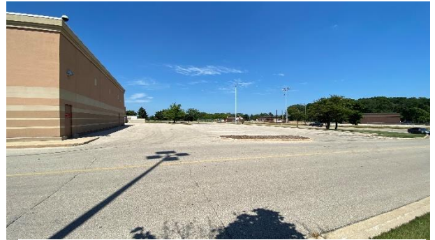
Looking at parking area east of store
