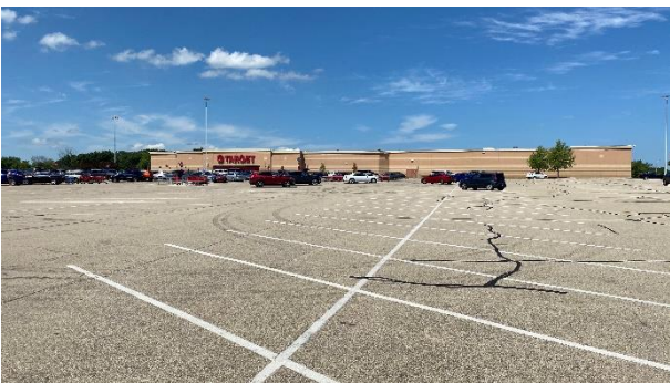
Looking north at existing store façade from parking area
