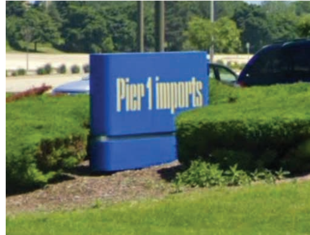
remove & replace existing sign
