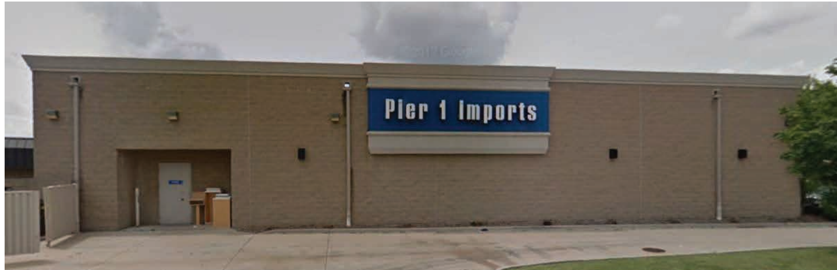
remove & replace existing letters [east elevation]
