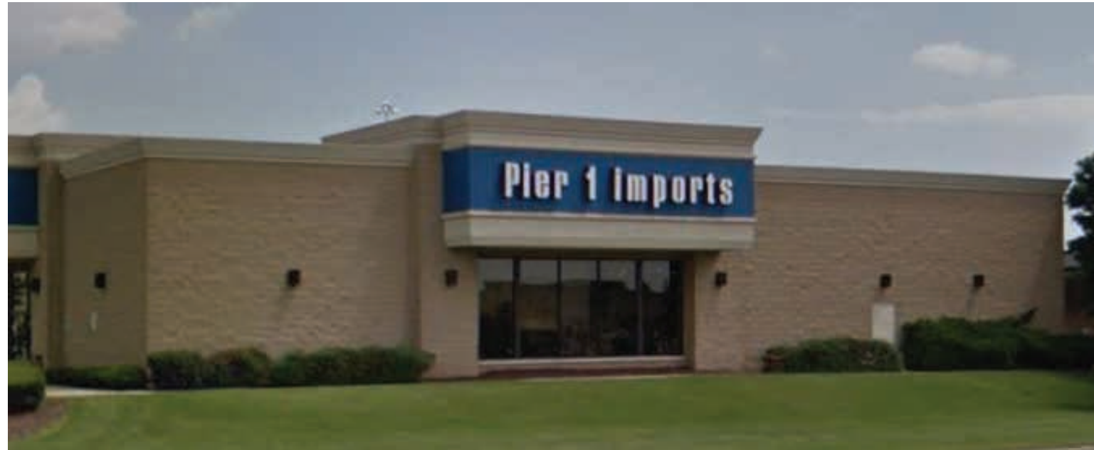
remove & replace existing letters [west elevation]
