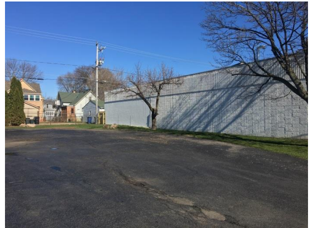
Looking northwest at west wall of subject property/building
