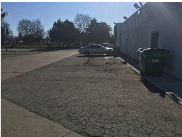
Looking east towards West Blvd from parking area of subject property
