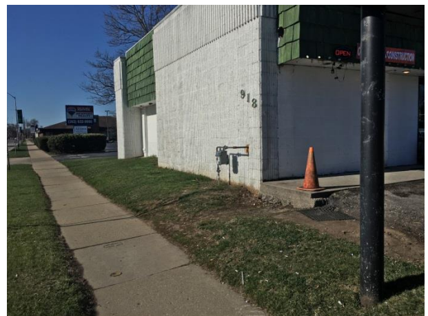
Looking south along sidewalk for West Blvd. Subject property to the right
