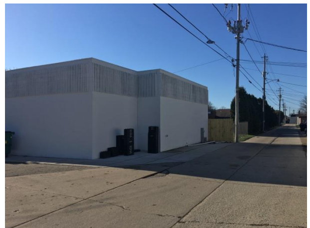
Looking south down alleyway at rear of subject property
