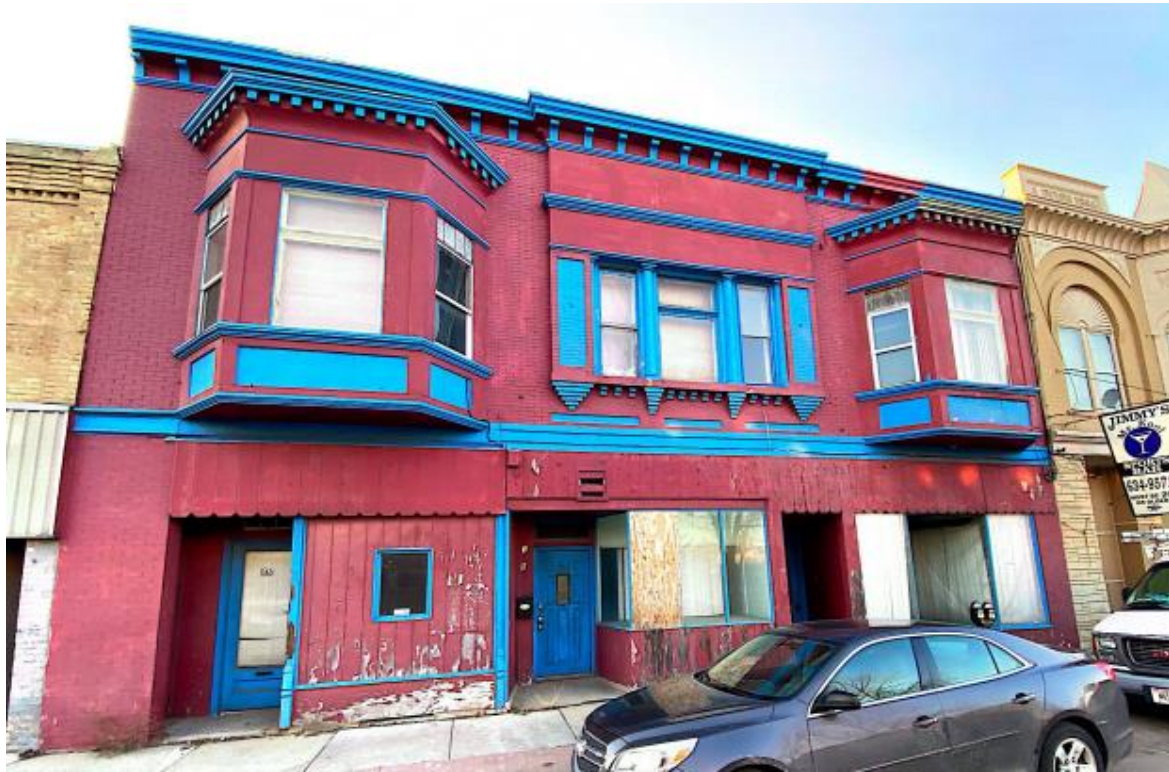
Current façade of 1334 Washington Avenue, picture provided by the applicant.
