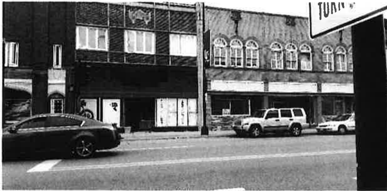
Building to the West of 1418-1424 Washington Ave.
