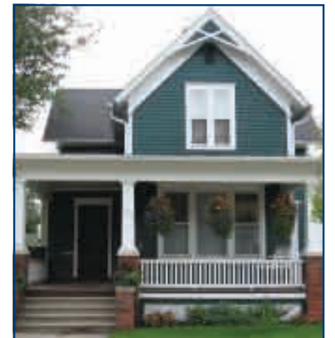
LEFT – The Community Oriented Policing House was custom designed with consultation from architects, historians, builders and police officers; TOP RIGHT – The Hernandez family stands on the porch of their new home on Racine Street. BOTTOM RIGHT – An attractive Tri Gabled Ell home on Park Avenue.
