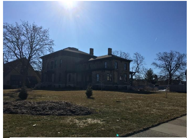
Looking southeast at the site from Kearney Avenue
