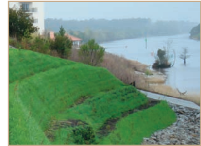
Another option to managing steep slopes or bluffs are living walls which offer eco-friendly erosion protection. A living wall is a vertical arrangement of vegetation that can help infiltrate stormwater runoff and prevent the soil from eroding. Photo courtesy of the Bruce Company.
