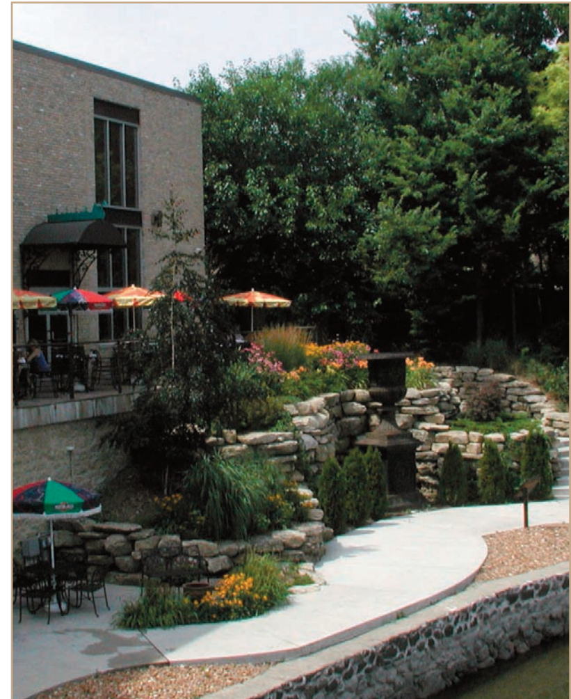
Example of riverbank stabilization and riverwalk in Fort Atkinson
