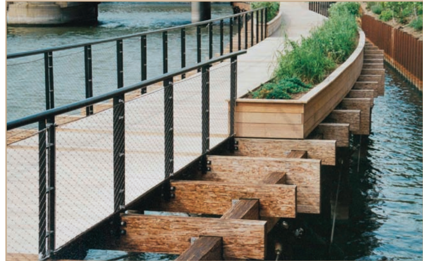
Example of cantilevered riverwalk treatment of Milwaukee Riverwalk.
