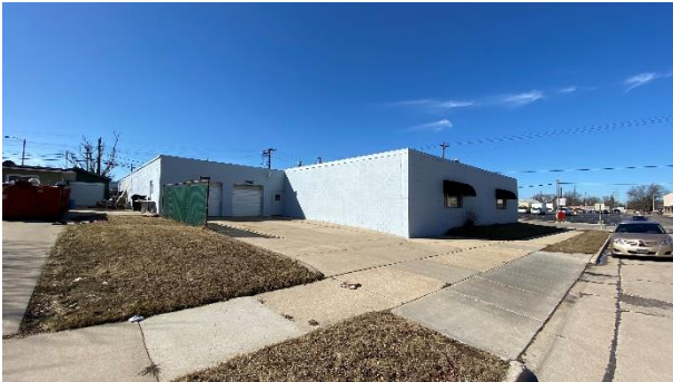
Looking northwest at site from Monroe Avenue
