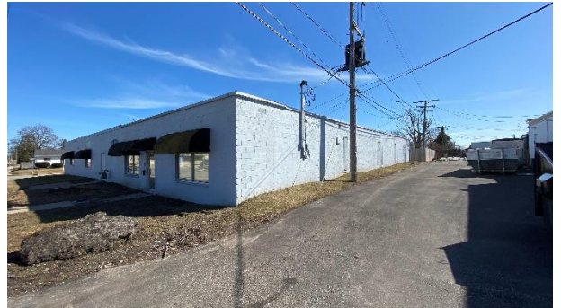
Looking southeast at site from 21 st Street
