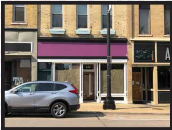
232 Main Street - Current View
