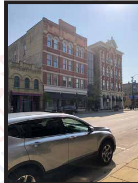
232 Main Street - Southeast
