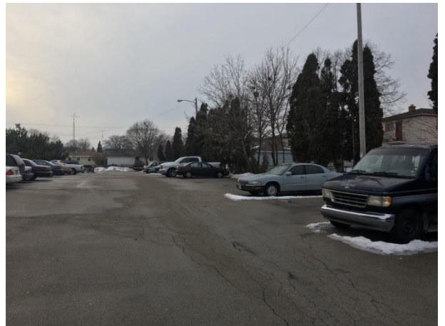
Looking (west) at rear of subject property
