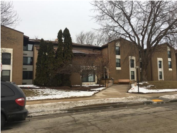
Looking north at subject property (middle of building)
