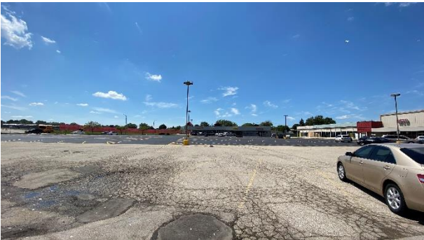
Looking west at the remainder of the storefronts in the center
