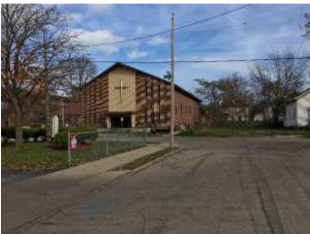
Looking east on Carroll Street from existing residential building
