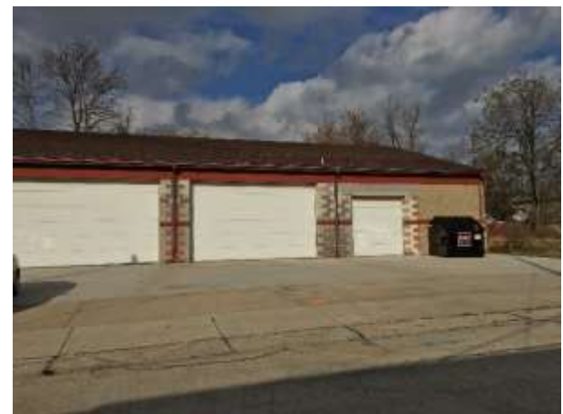
Looking north at existing garage, proposed for demolition
