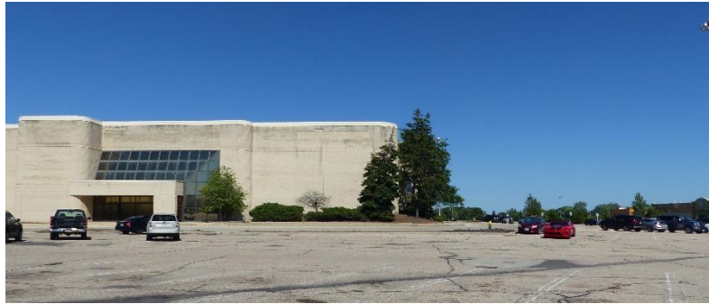
Looking east from subject property
