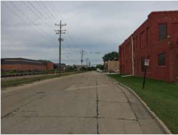
Looking north along Holborn Street, subject property to the right
