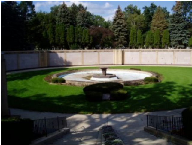
Lower Level Existing Crypts and Fountain
