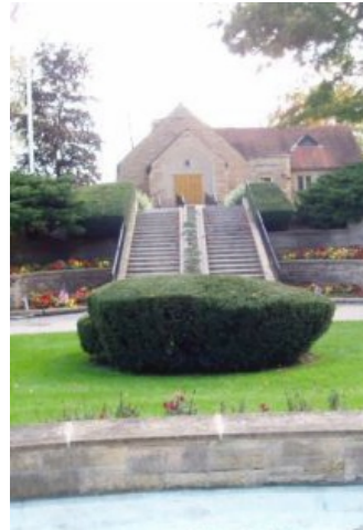
Stair to Upper Level
