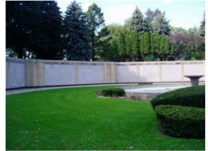
Existing Lower Level Crypts
