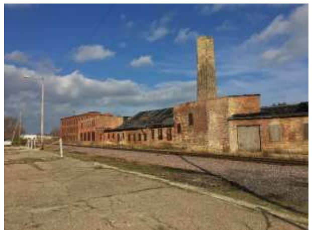
Looking at west side of property, adjacent to railroad right-of-way
