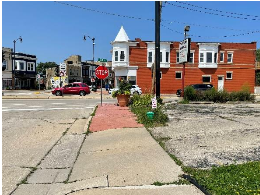
Looking across the street from subject property
