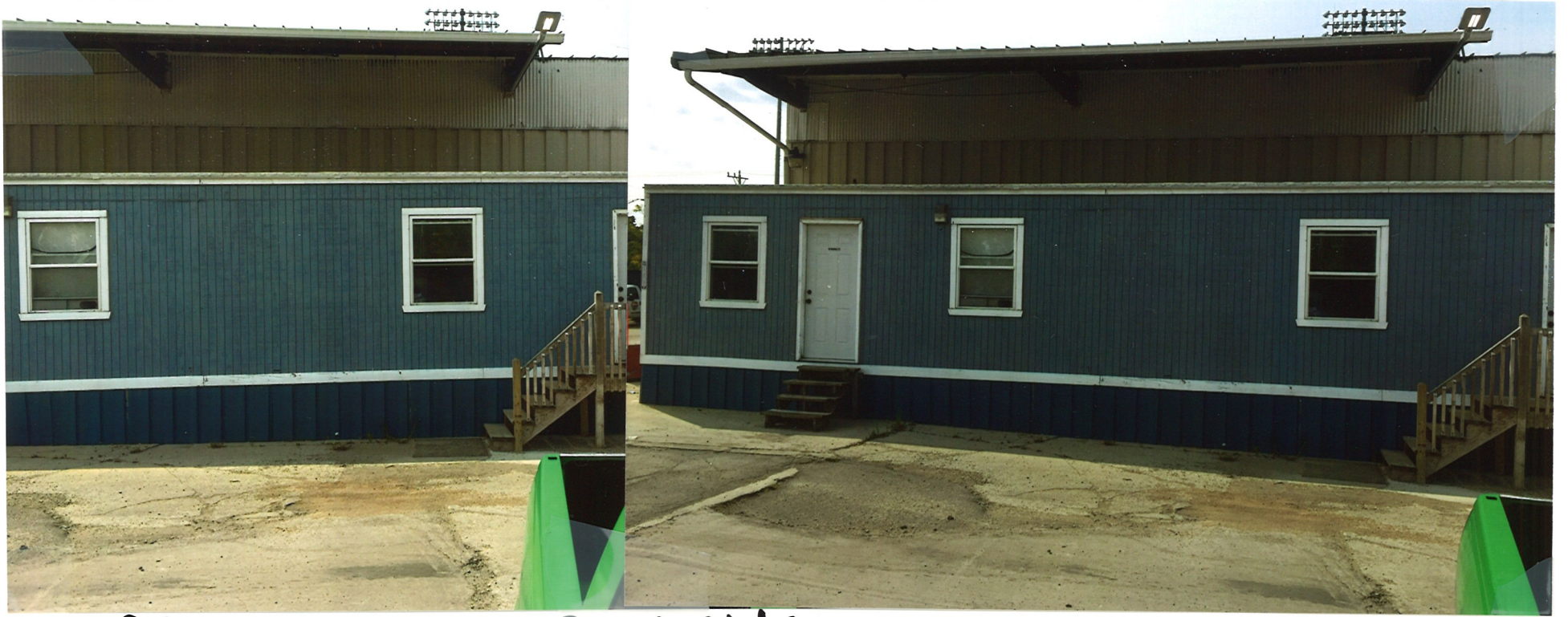
Office Trailer - East side
