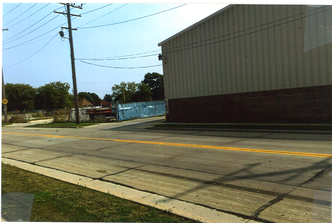
North Side of Bldg
