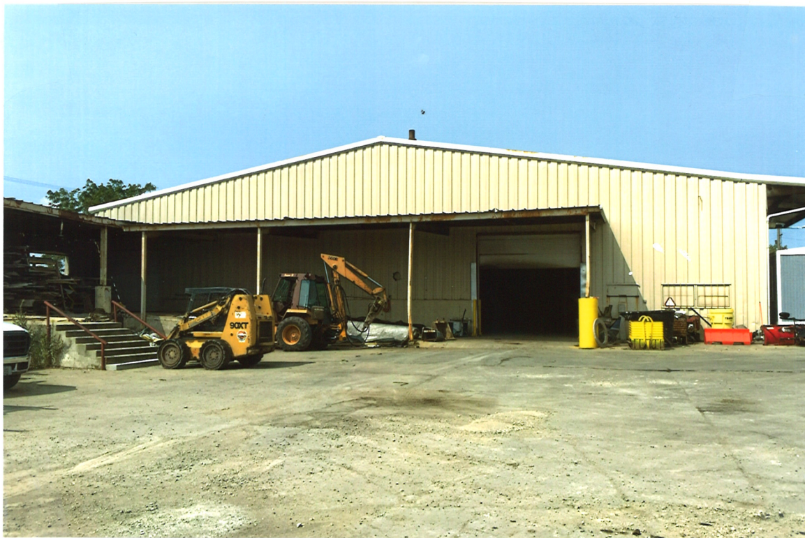
South Side of Bldg
