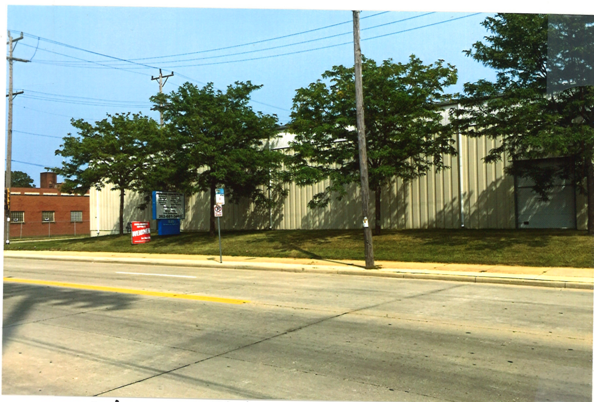
West Side of Bldg
