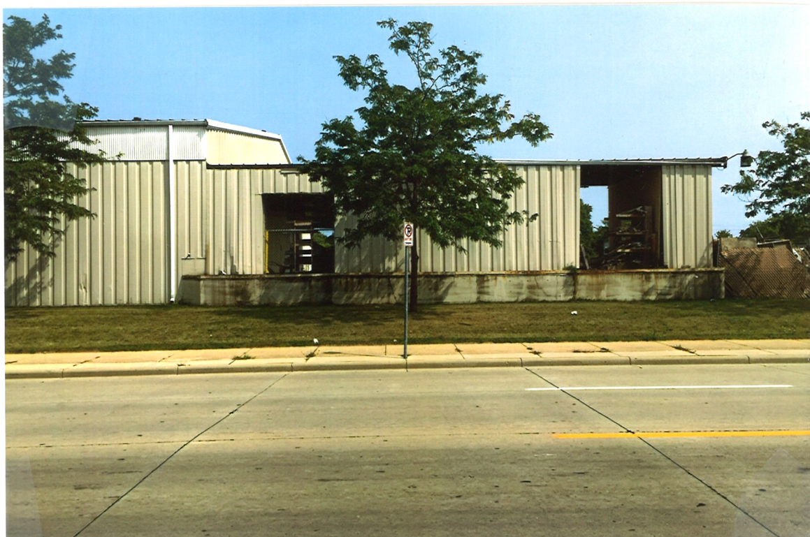
West Side of Bldg
