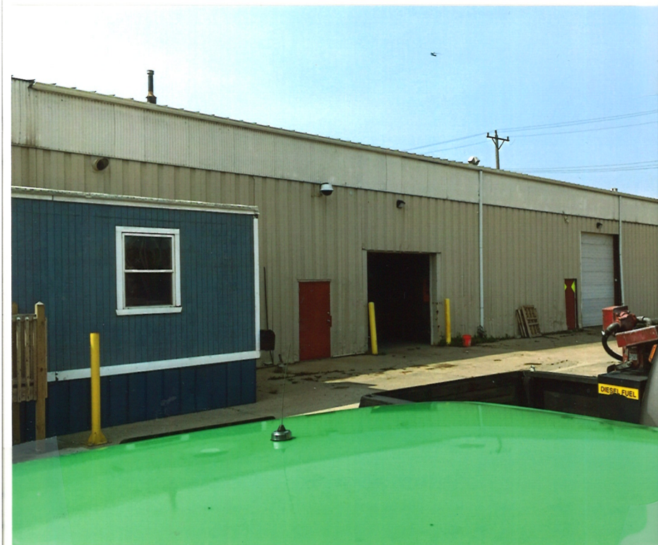
East Side of Bldg
