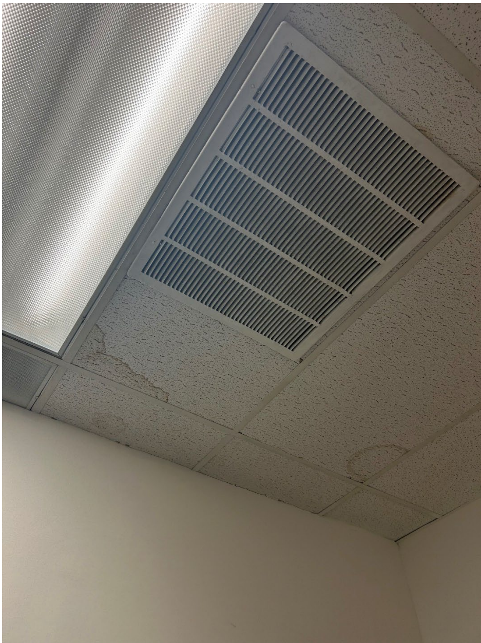
Water damaged ceiling tiles
