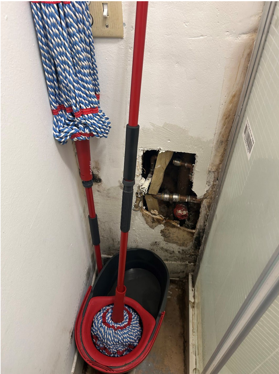
Bathroom- hole in wall, suspected plumbing leak
