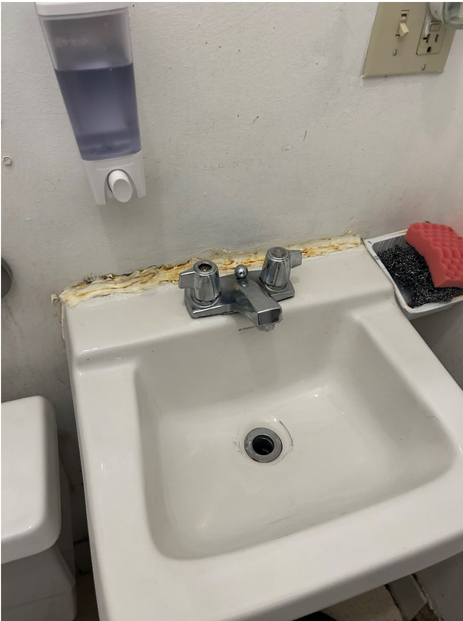
Caulk in disrepair at bathroom sink
