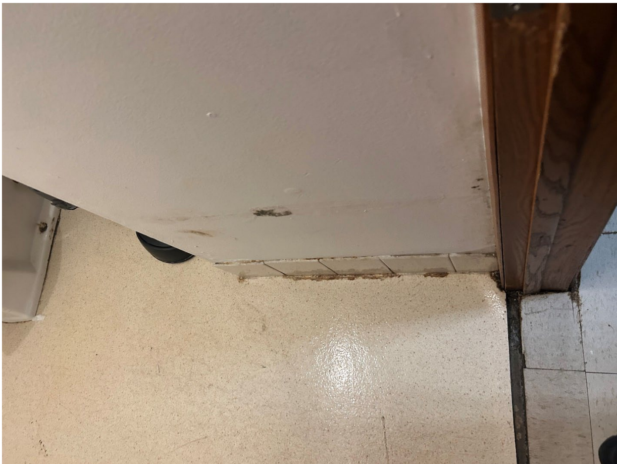
Bathroom- soiled wall, missing door threshold, base coving in disrepair
