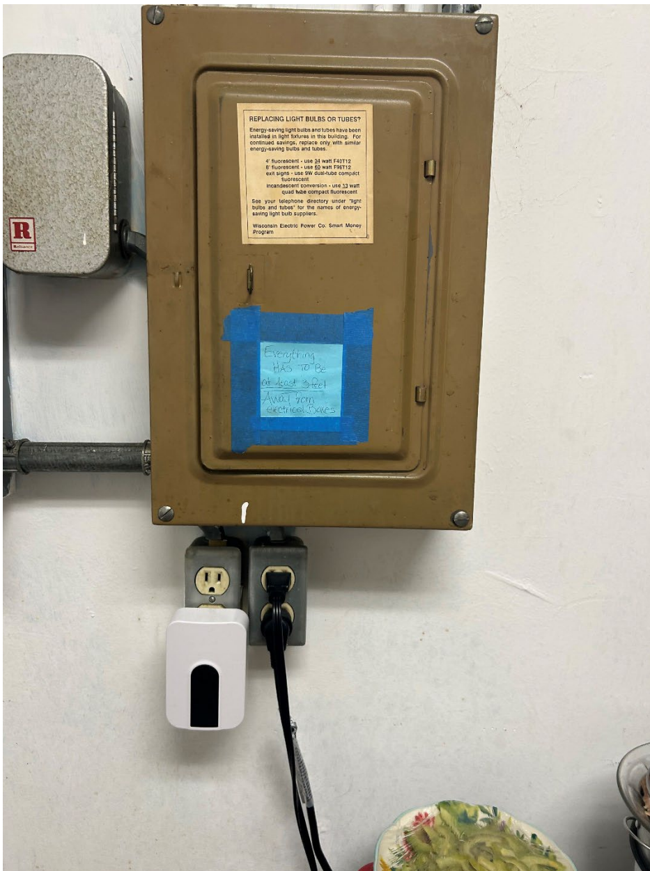
Electrical box above kitchen prep space with note stating, "Everything has to be at least 3 feet away from electrical box"
