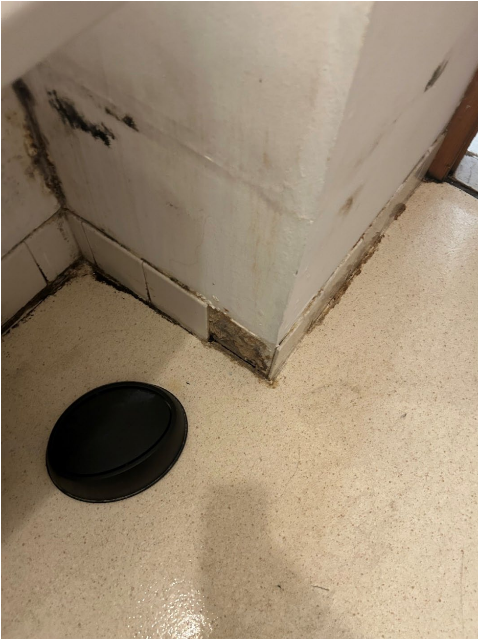
Water damage in bathroom & missing base cove
