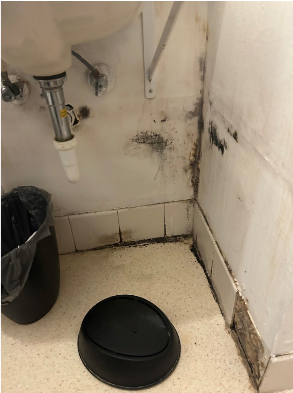
Water damage in bathroom & missing base cove
