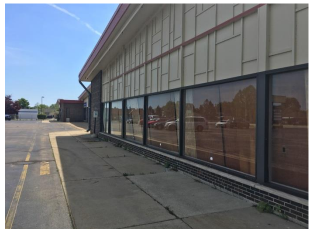
Looking east at building where Daycare would be located
