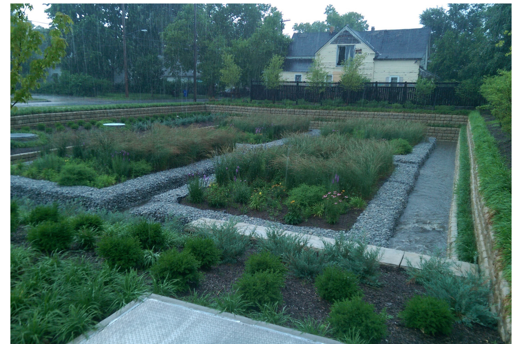
Fleet Avenue Green Infrastructure, Cleveland, Ohio
