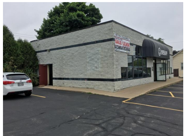
Looking northwest at subject property
