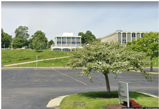
View looking west from Pershing Park Drive
