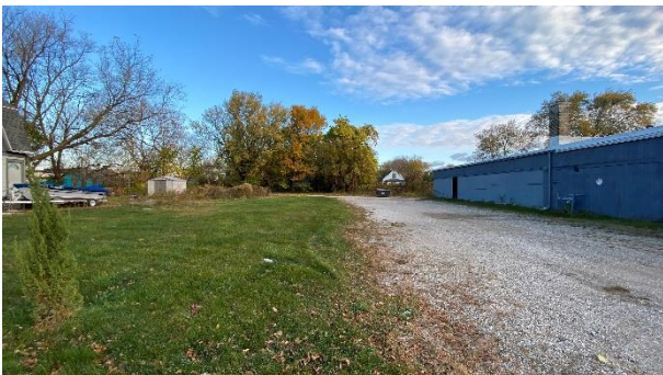
Looking at west side of building
