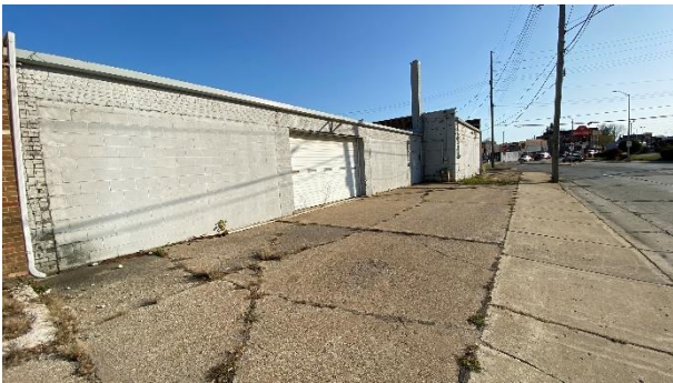
Looking at west side of existing building on the property
