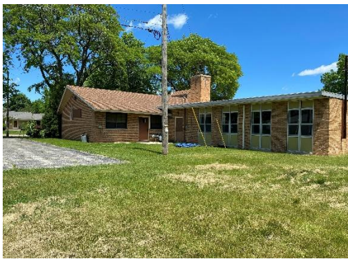
Looking Northeast at site
