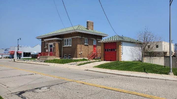
Looking at the South and West of the Building
