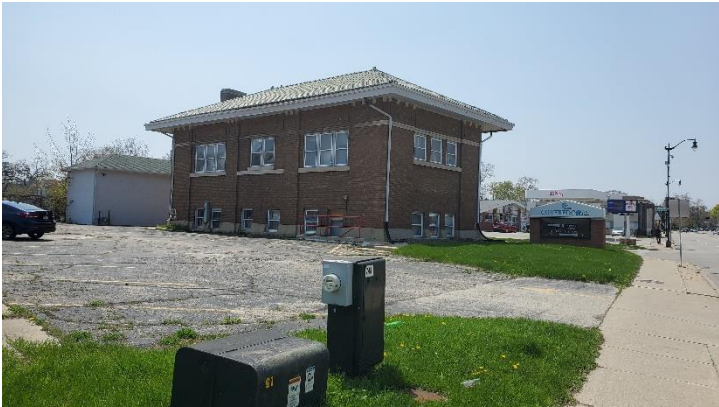
Looking at the North and East of the building.
