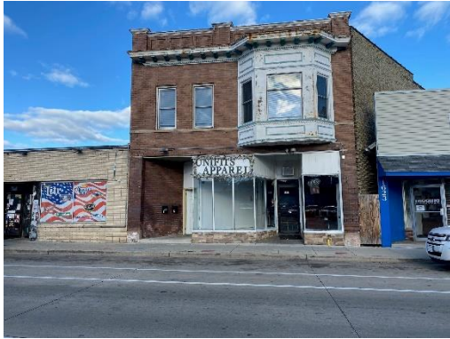
Looking east at subject property
