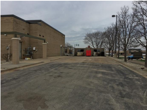
North side of subject property with trash handling area and loading zone
