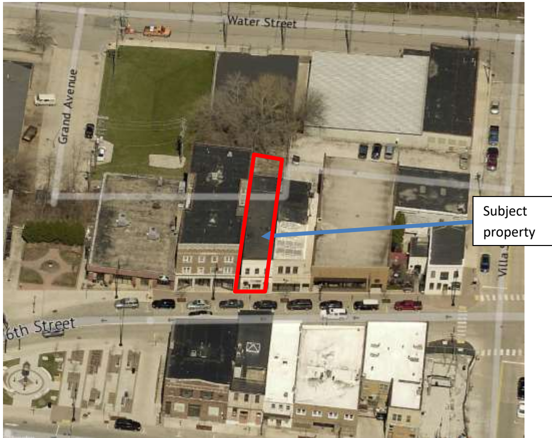
Birdseye view of the building, indicated in red (image from City Pictometry)
