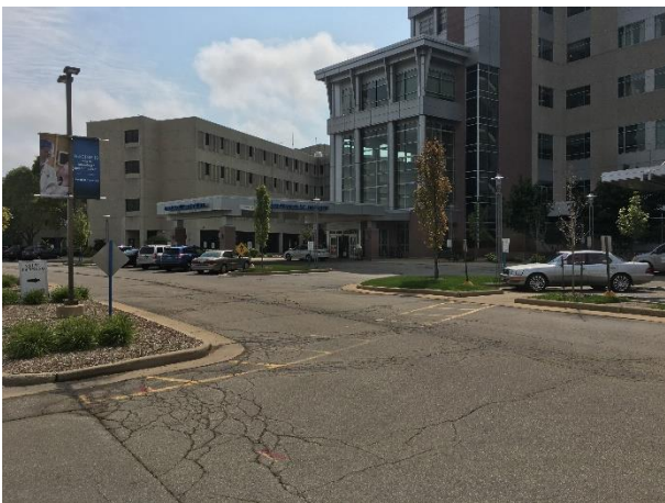
Looking southerly from parking lot of subject property at main hospital building
